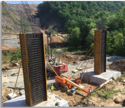
Pier formation for bridge 6 over Little Scioto River Seg 1/2a
