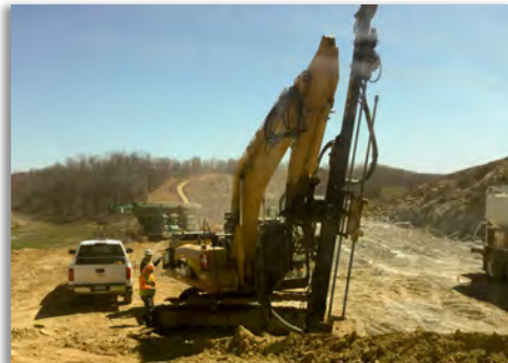
Drilling rig drilling for pre-split blast Seg. 3b
