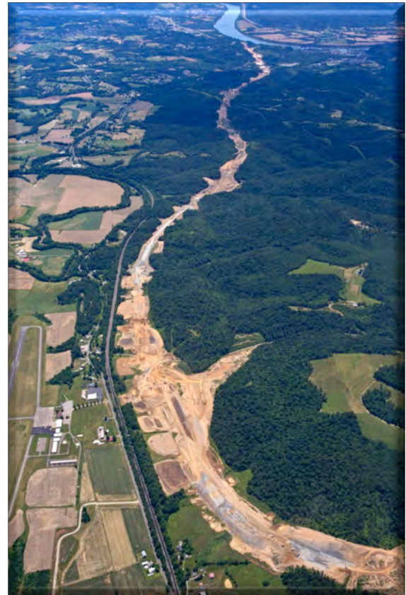
Shumway Hollow interchange looking south toward U.S. 52 June 2016
