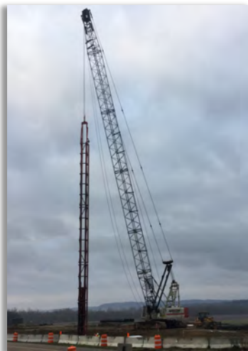
Pile driving for bridge abutment Seg. 4
