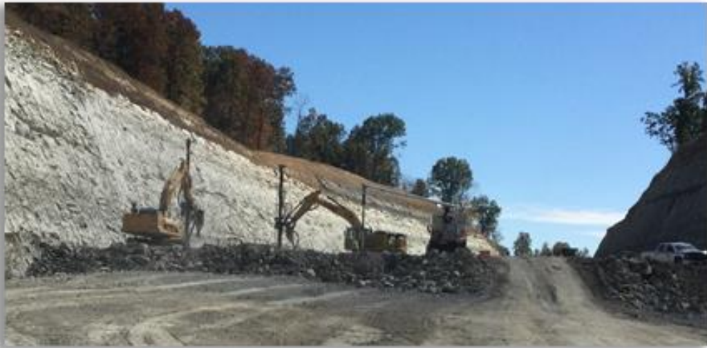
At left are rigs drilling blasting holes for production blast in Segment 3B of the corridor.
